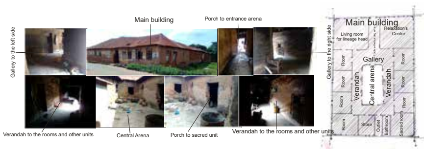
Plate 1: Exterior and Interior Structures with Drawing plan of Yorùbá Architectural Compound Town: Ara, Year of Photographs: 2021 Arrangement and Drawing: Ajadi Michael Olaniyi
