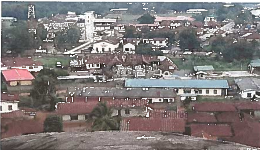
Figure 1. Aerial view of the Ògògà Palace and the surrounding community. Photo credit: Arc. Ablodun Bamidele.
