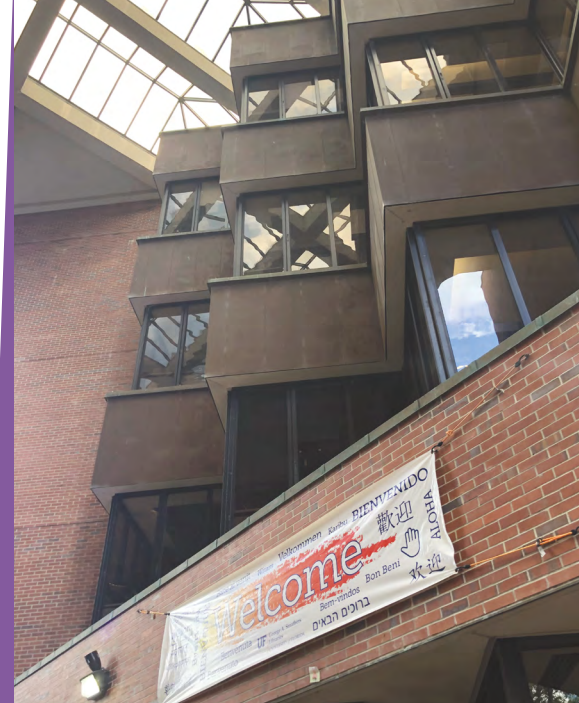
Above: View from Turlington Plaza with iconic design of the third, fourth, and fifth floors.
