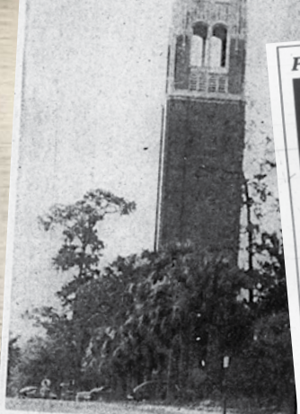
FINALLY COMPLETED in the interim between spring and summer terms, the Century Tower bears out supporters' forecast that the costly structure will be seen from any spot in surrounding territory. Viewed here from Newell Drive, the red brick tower raises its long-awaited cap above the trees past Stadium Road. Next stop: finishing the interior.
