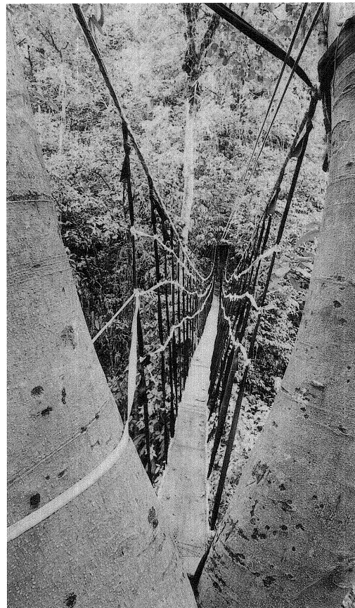
→ FIGURE 1. Two views of the completed walkway looking east from the strangler fig tree toward the hillside entrance.
