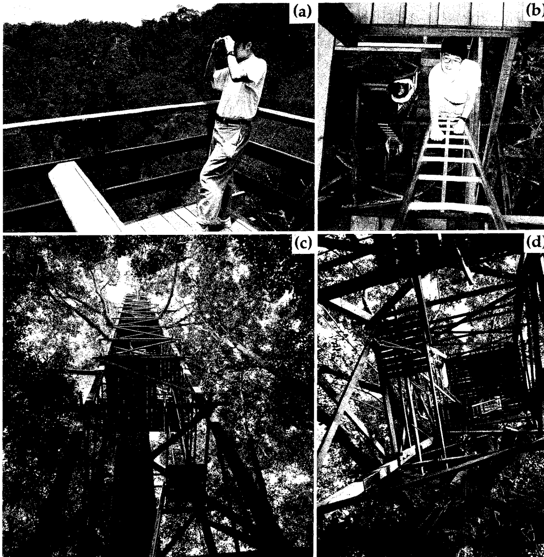
FIGURE 5. Tree Tower 2 (T2). (a) the top platform, (b) climbing up to the top platform, looking down from there, (c) a total view of T2, (d) an inner view of T2.
