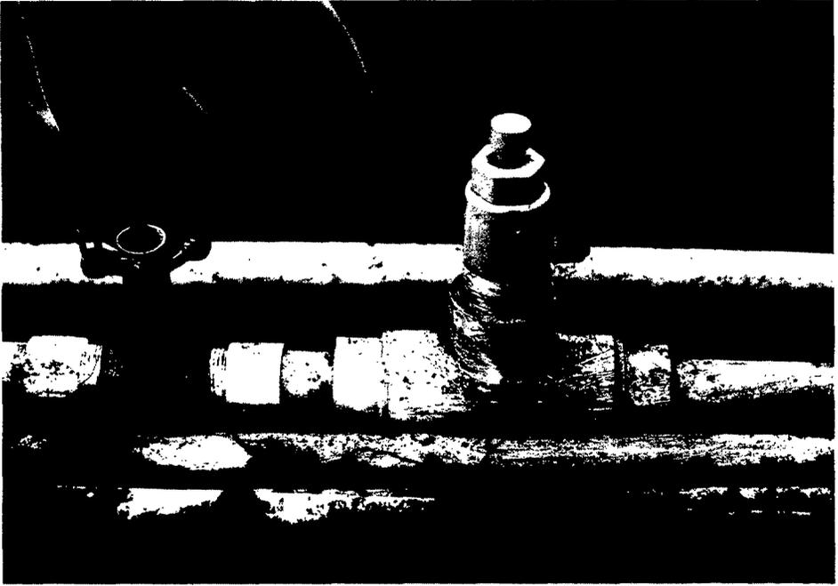
FIG. 6. Gate valve for an individual manifold, with a vacuum breaker equipped with a pressure valve for checking water pressure to an individual treatment replication (right).
