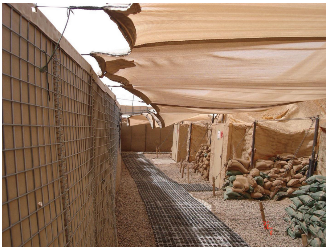
Figure 1. A HESCO perimeter at a US military outpost in southern Iraq, 2009. The HESCO wall is seen on the left and in the far background. A narrow walkway separates this structure from tents and other living areas to the right.
