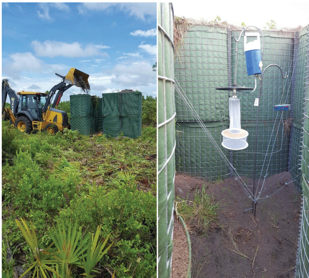
Figure 2. One of 16 two-tiered HESCO perimeters under construction at Camp Blanding Joint Training Center, Starke, FL (left hand image). Access door made of two stacked side panels from a broken-down HESCO MIL cell is visible at left front of this perimeter. Right hand image shows placement of a CDC light trap baited with dry ice to sample mosquito populations inside a soil filled HESCO perimeter.
