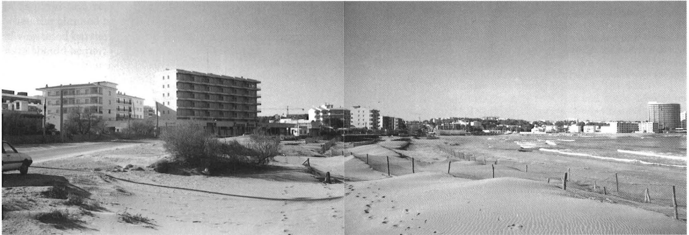
Figure 6. Alignment of nylon mesh fences installed parallel to shoreline and approximately perpendicular to the predominant winds blowing from the northern sector.
