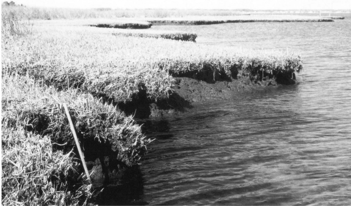
Figure 3. View of the Horse Island marsh shoreline illustrating the erosional scarp and the rootmat overhang. Note that the marsh neck next to the meter stick in the foreground is beginning to topple due to excessive undercutting.
