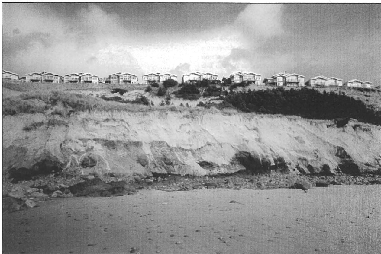
Figure 4. The Capes development north of the Netarts Bay inlet. Erosion cut away the toe of the cliff, re-activating a large landslide upon which the development had been placed (Photo: Komar).
