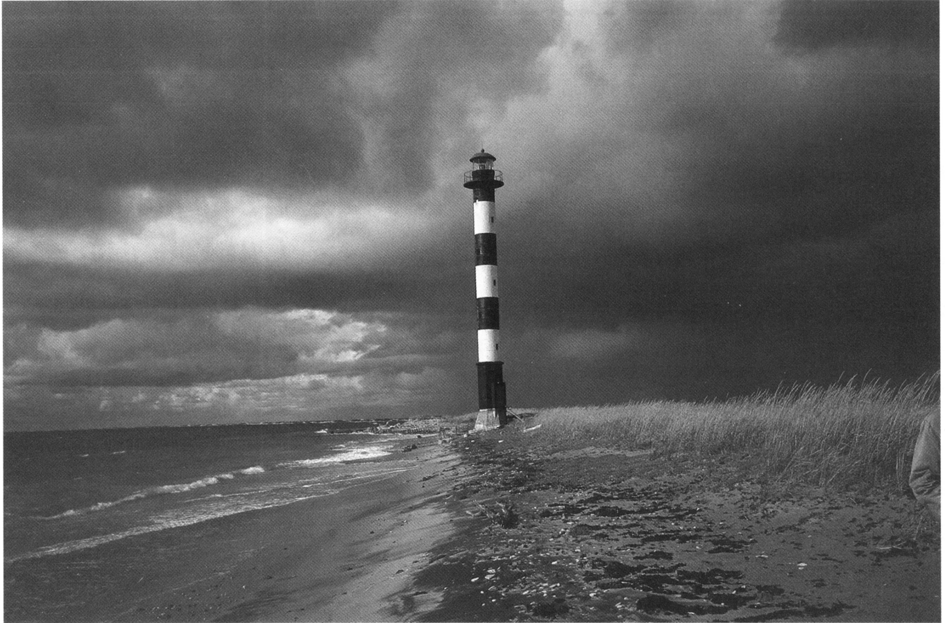
Lighthouse at the Kiipsaare cusplate spit on Saaremaa island in the Baltic Sea northwest of mainland Estonia. When built in 1931 the lighthouse was located 30 meters from the back of the beach, in 1981 it was 5 meters from the beach, and at present much of the foundation is exposed on the upper foreshore. (Photo: Maury Schwartz. Taken Sept. 10, 1991, four days after Estonia regained its independence.)
