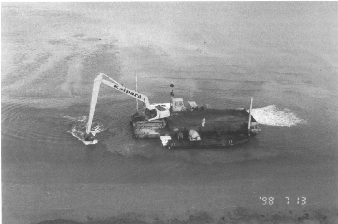
Figure 3. The dredging of muddy sediments from the marina approach channel using a digger mounted on a barge.
