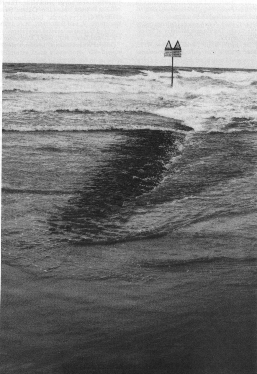
PHOTO 186. Locally supercritical longshore current. It is difficult to infer motion of longshore currents from one photo, but here a low groin acts as a broad-crested weir over which the longshore current turns supercritical as it flows from left to right. On the downstream side of the groin, the current goes through a hydraulic jump, reverting to subcritical flow on the right. The groin consists of fitted basalt blocks ( cf. PHOTO 185 on page 1012), a typical Dutch construction, at Scheveningen, The Hague, on the Dutch North Sea coast. (Photo: Cyril Galvin, Box 623, Springfield, VA 22150). [Photo taken 9 July 1990]
