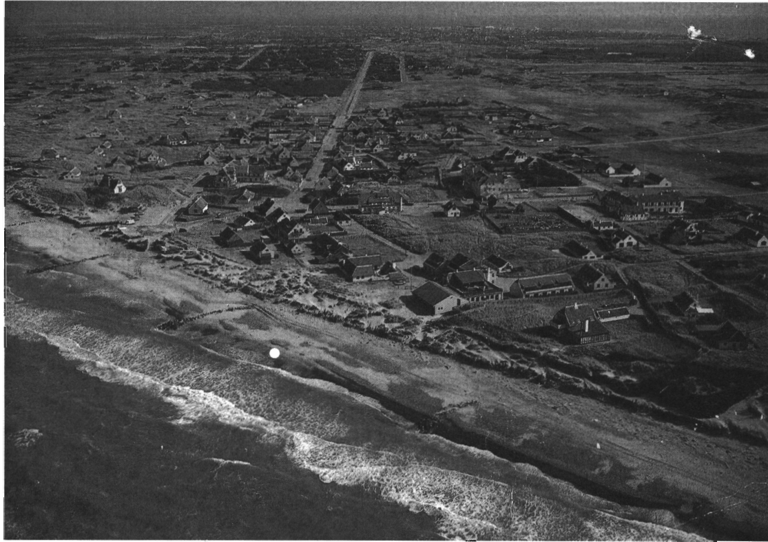
Figure 2. Groins at Gl. Skagen, 1960.
