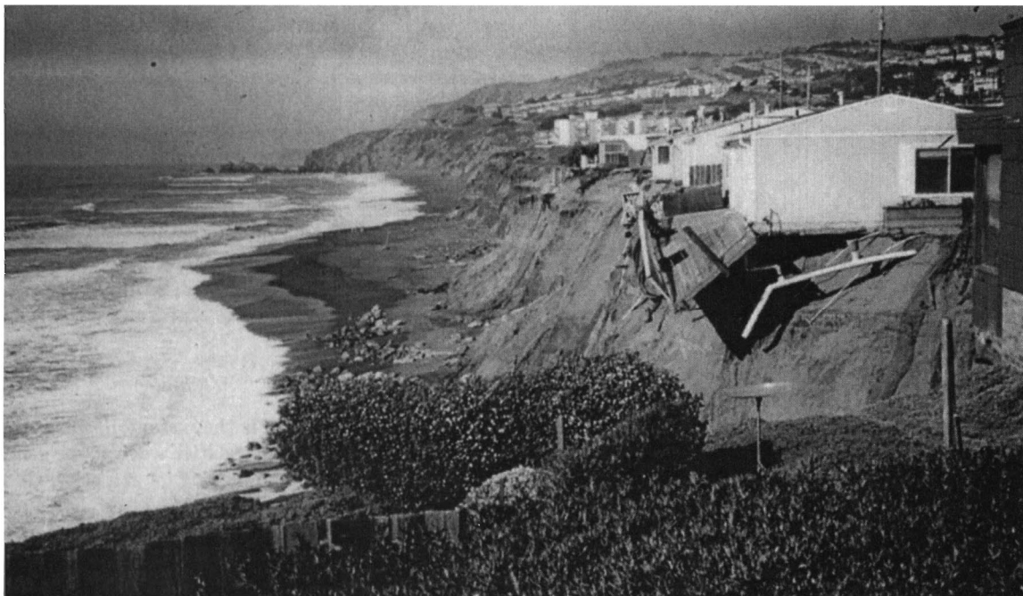
Figure 4. Erosion of the seacliff and undercutting of houses along the Esplanade at Pacifica in March of 1998. Rip-rap on the beach marks the location of the cliff toe before the winter storms. The scatter of these several-ton boulders testifies to the wave energies encountered along this section of the central coast during the 1997–98 ENSO storms. Photograph courtesy of Monty Hampton, U.S. Geological Survey.
