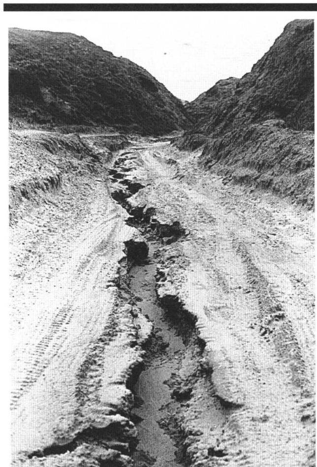
Figure 14. Artificial road gap, hewn at right angles to the cliff, repeatedly eroded, re-excavated and re-eroded.
