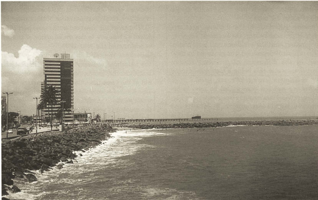
Figure 7. Waterfront at point 5 looking to the west showing a revetment and the absence of a beach.
