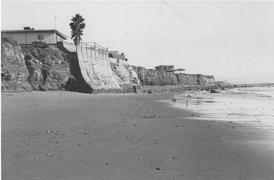
Figure 5. Two contiguous 6-m-high 21 and 23 m length sea walls near El Sauzal showing significant differences in design and construction procedures. Beach width in front of structures is 12 m to the wet area.
