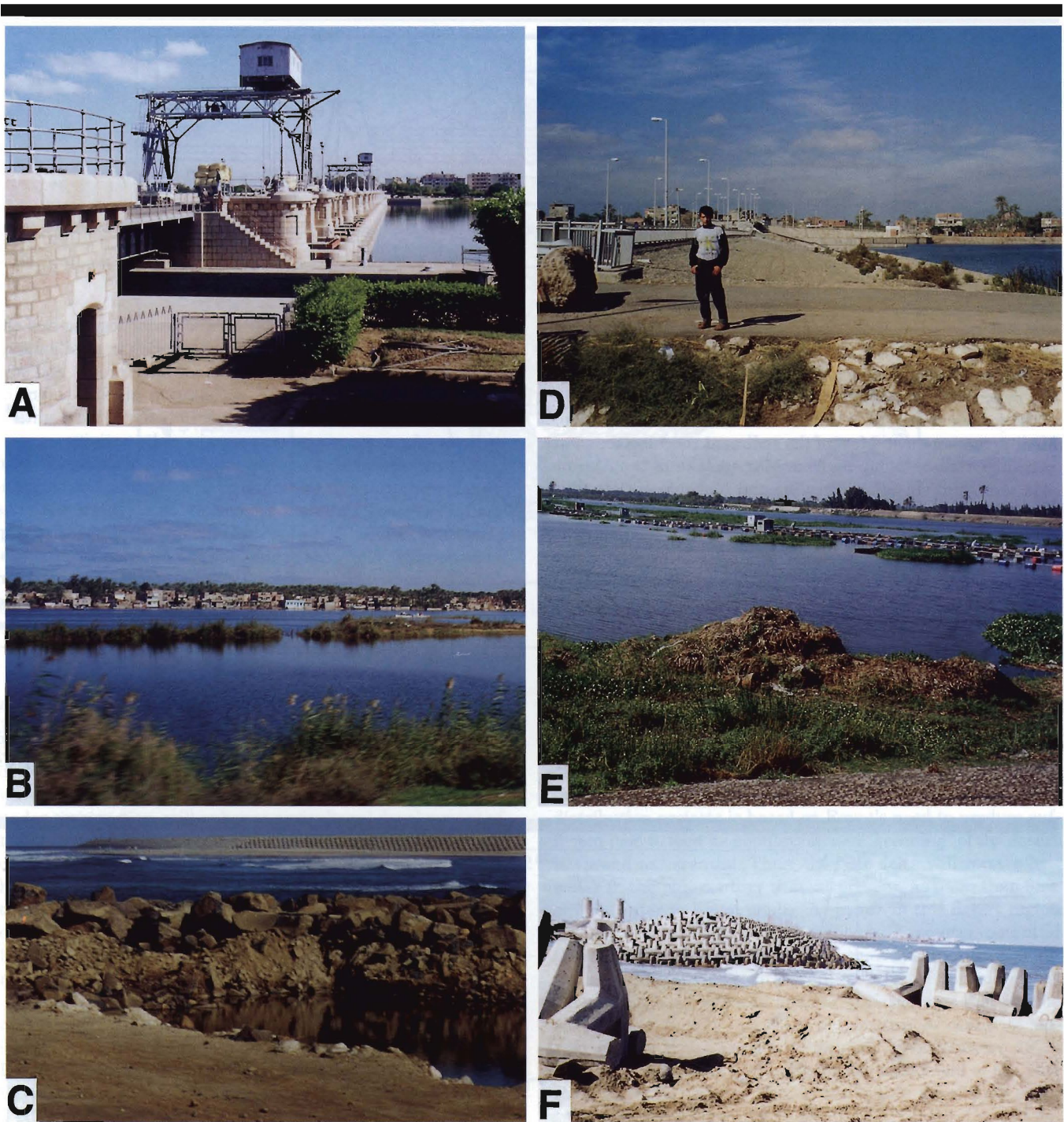
Figure 16. Photographs, taken in November 1997, showing human modification of the Rosetta and Damietta distributaries of the Nile in northern delta. (A) Edfina barrage, view towards NE (Figure 15); (B) vegetated islands forming in the Nile channel below Edfina, view towards ENE; (C) sea water entering the mouth of the Rosetta branch as shown by landward-driven waves, view towards NE; (D) Faraskur Sudd barrage, view towards NW; (E) vegetated islands and fishing huts in river channel just below Faraskur Sudd barrage, view towards W; and (F) artificial structures emplaced to protect rapidly eroding coast at the Damietta promontory, east of Ras El-Bar (in distance), view towards W.
