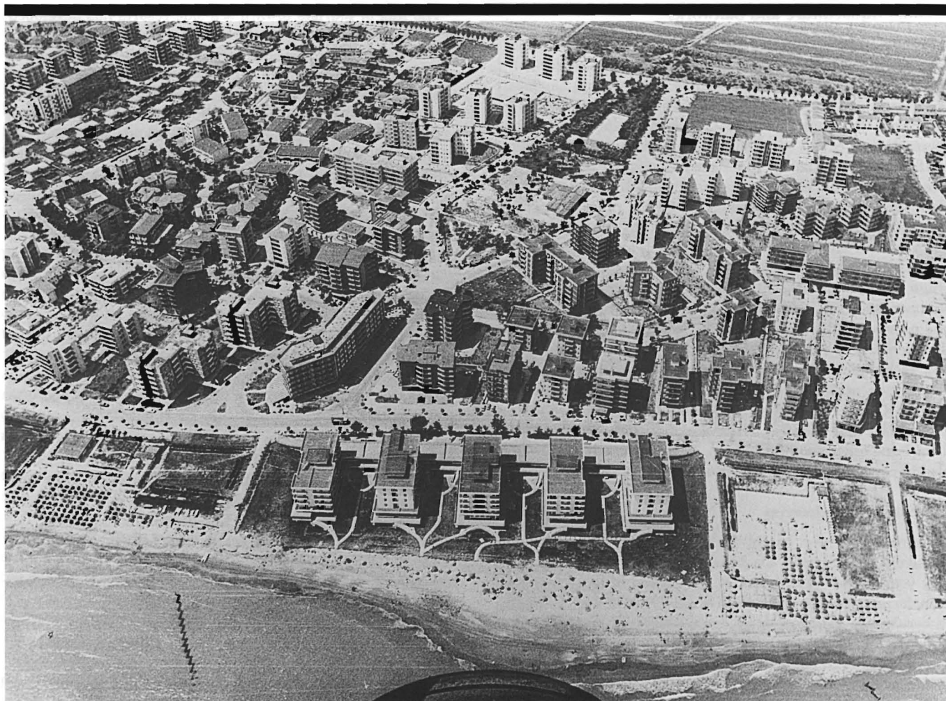
Figure 12. Heavy concentration of buildings behind the shoreline at Lido Adriano, south of the Po delta.
