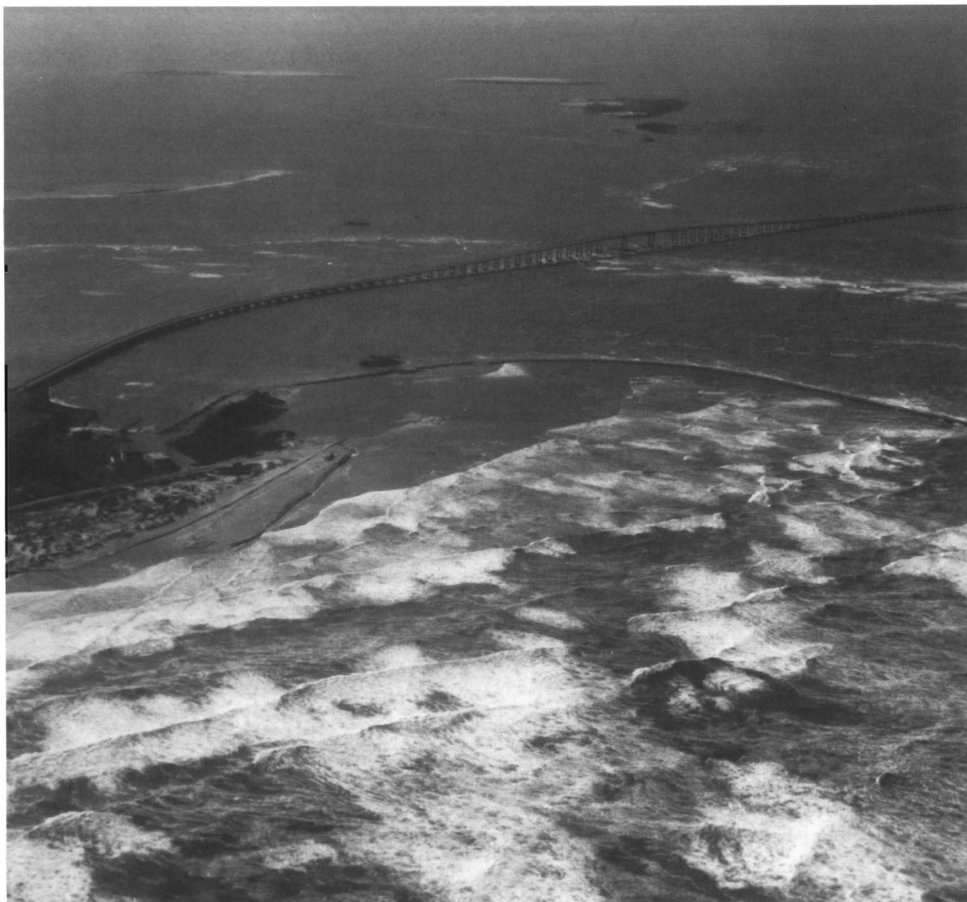
Terminal Groin at Oregon Inlet, North Carolina. View looking west on 31 October, 1991 during the height of the "Halloween" storm when the significant wave height was 5 m with associated periods of 22 sec. The Terminal Groin (foreground) was constructed by the NC Dept. of Transportation as an emergency measure to protect the Bonner Bridge and its abutment to the north end of Pea Island. The structure met the challenge of a barrage of extremely severe storms during the Fall of '91 and Winter of '92. (Photograph by Carl Miller, WES/CERC Field Research Facility, Duck, North Carolina).
