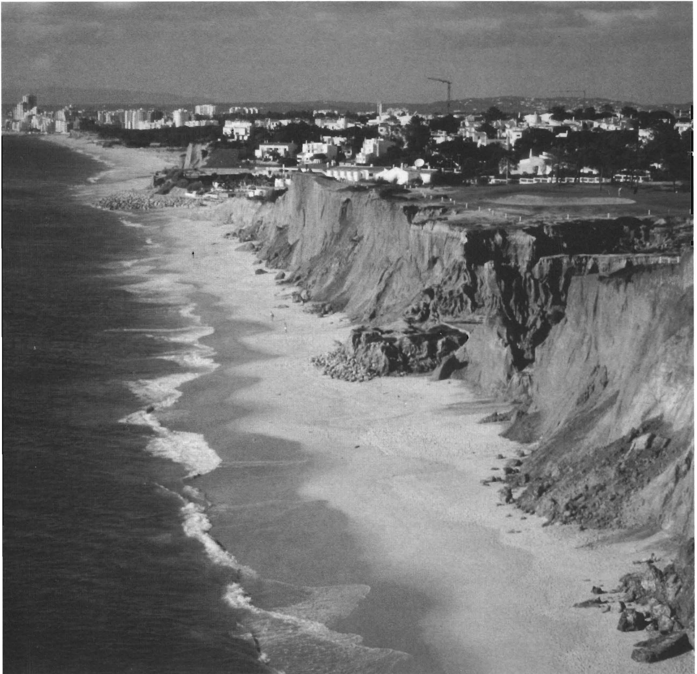
Rapid cliff erosion on the Algarve coast, southern Portugal. Vale do Garrão riprap protrudes seaward at the base of the flanking cliffs. In 1984, the cliffs were at the position of the riprap. Inland displacement of the beach is seen at the top of the photo, towards Quartiera. (Photo: João Alveirinho Diaz, Instituto Hidrografico, Lisbon, Portugal).
