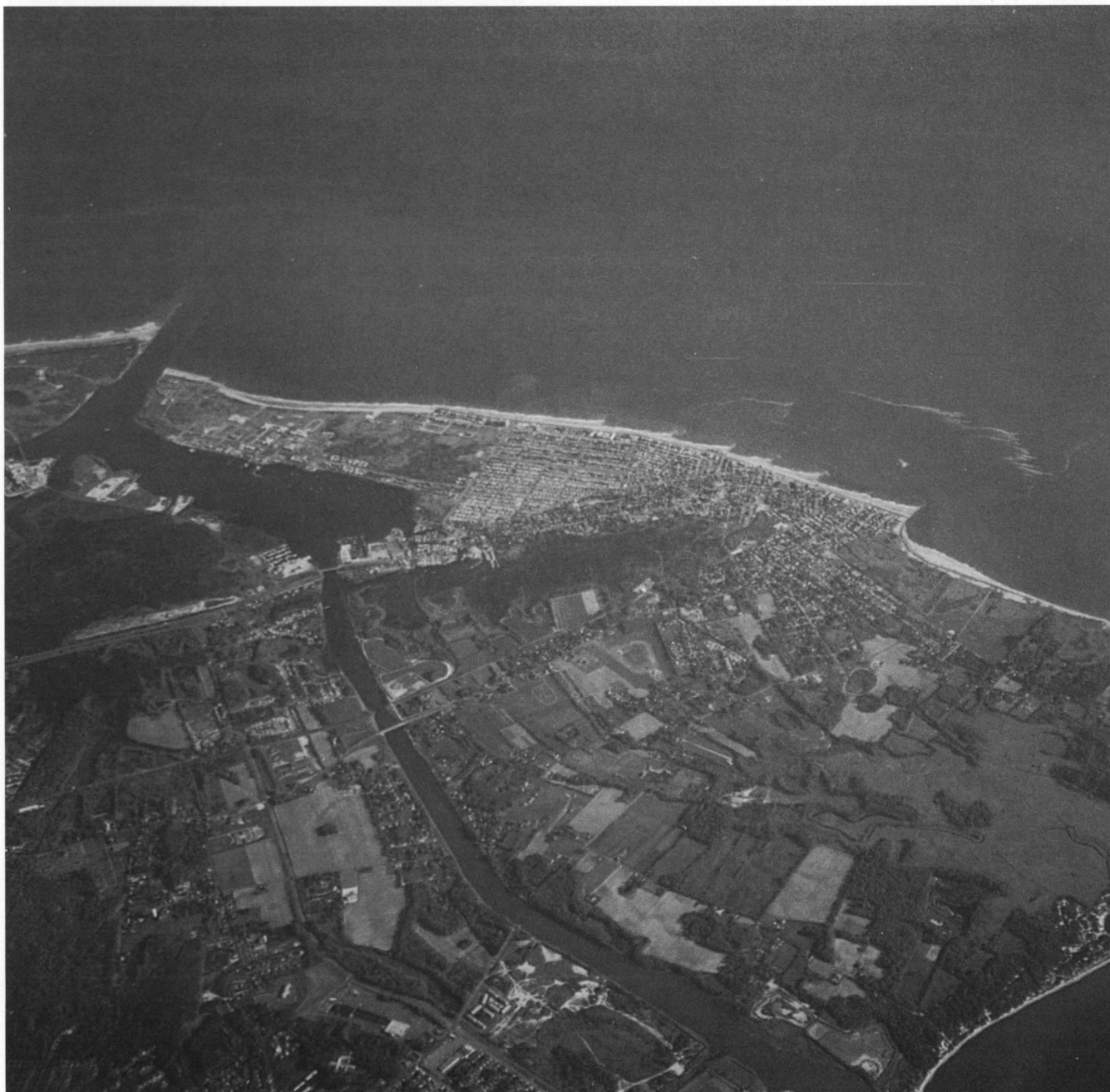
Cape May, New Jersey. Jetties at Coldspring Inlet in the upper left of the photo have caused an offset in the shoreline. A groin field protects the shoreline of the City of Cape May in the center of the photo. (October 29, 1991 by Fred E. Camfield, Wave Dynamics Division, Coastal Engineering Research Center, US Army Engineer Waterways Experiment Station, Vicksburg, Mississippi).
