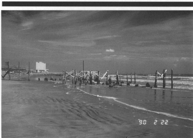
Figure 7. 1990 Folly Beach with remains of pier.
