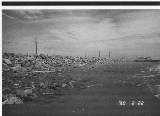
Figure 15. 1990 Folly Beach looking northeast and showing large rubble revetment in hot-spot area water line in far right of photograph.
