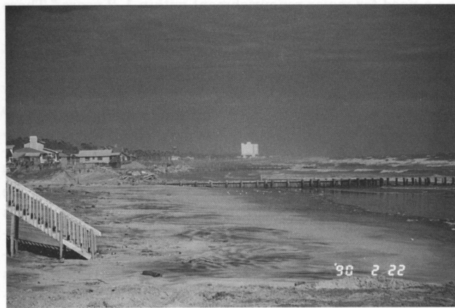
Figure 5. 1990 Folly Beach with rubble and erosion up to structures.
