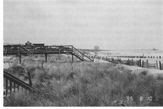
Figure 6. 1995 Folly Beach fill corresponding to Figure 5. Extensive vegetated berm and wide beach.
