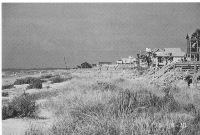
Figure 10. 1995 Folly Beach fill corresponding to Figure 9 and showing wide vegetated berm and beach.
