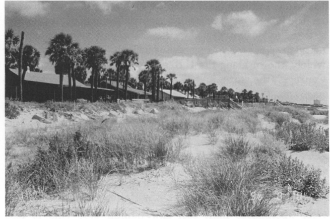
Figure 4. 1995 Folly Beach fill corresponding to Figure 3. Extensive vegetated berm.
