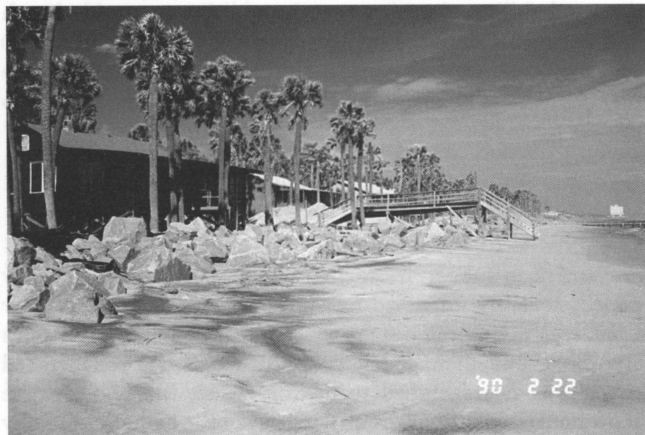
Figure 3. 1990 Folly Beach with rubble revetment.
