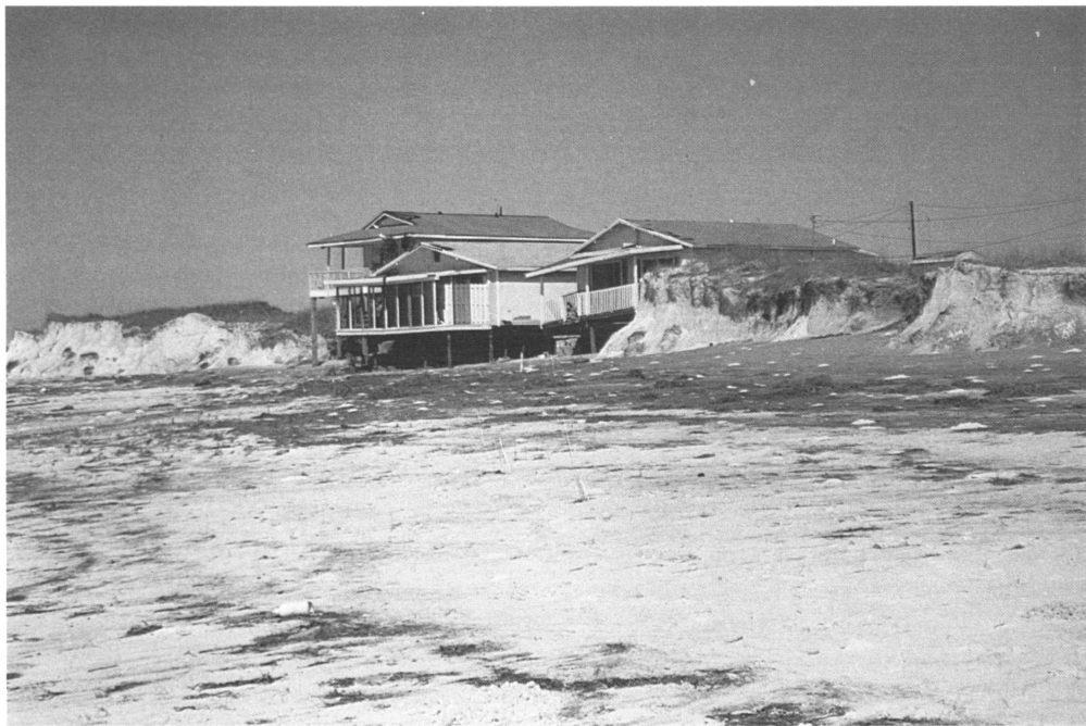
Figure 3. These houses west of Hollywood Beach illustrate the impact of removing dunes. Despite being elevated slightly and set back approximately 60 m from the shore, prior dune removal resulted in some structural damage to these single family homes during Opal. Had the houses been built behind the dune, damage would have likely been minimal.
