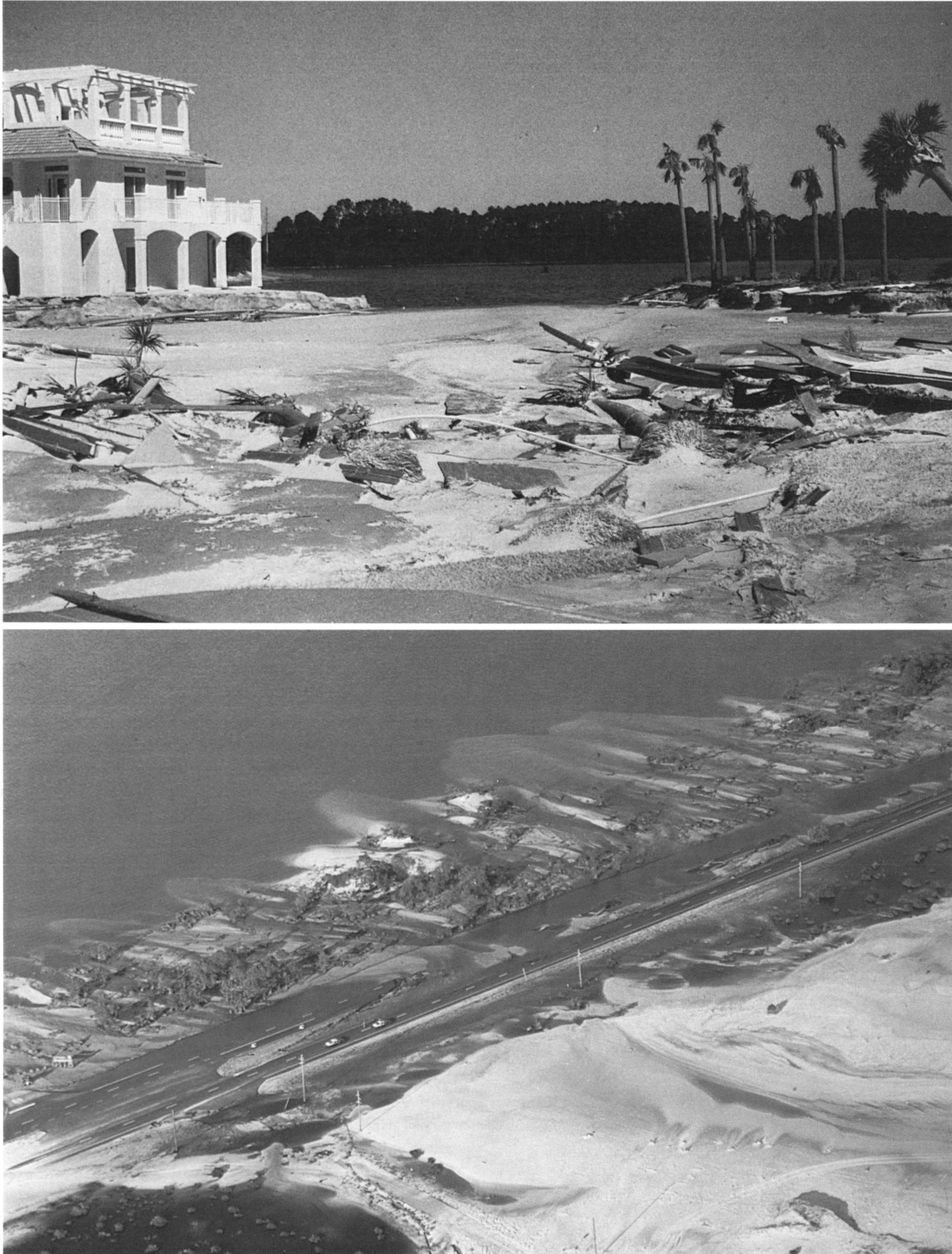
Figure 8. Storm surge flood scour occurred in many areas. By their nature, these areas are prone to repeat flooding and should be noted for future development restrictions. 8A. Channelized overflow of this area near Destin resulted in intense storm surge flood scour. 8B. In Fort Walton Beach, overflow scoured away Florida Route 98 and deposited washover fans in the lagoon.
