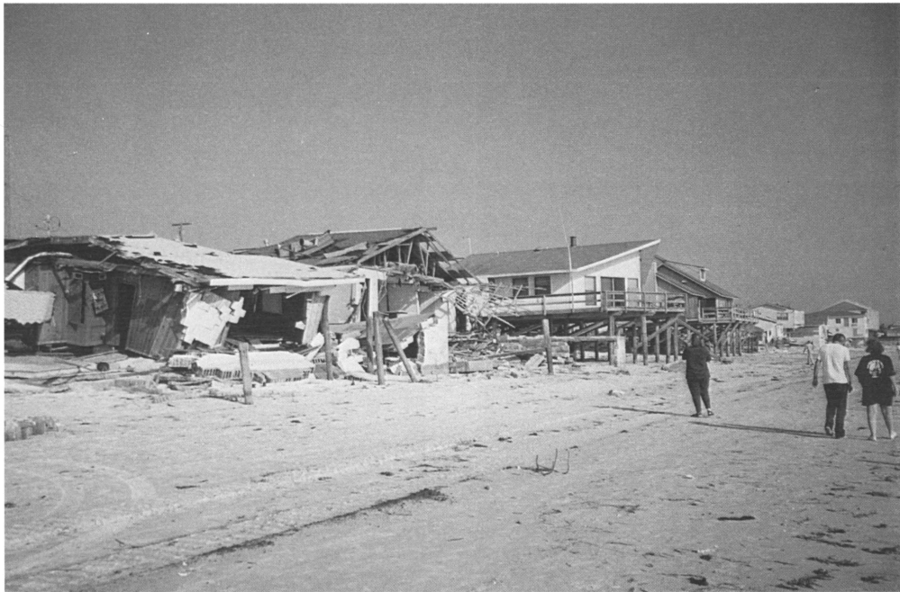
Figure 2. The importance of building above grade is shown by these four single family homes in Mexico Beach. The two on the left were built at grade and completely destroyed by storm surge, while the two on the right are elevated on pilings and suffered no structural damage.
