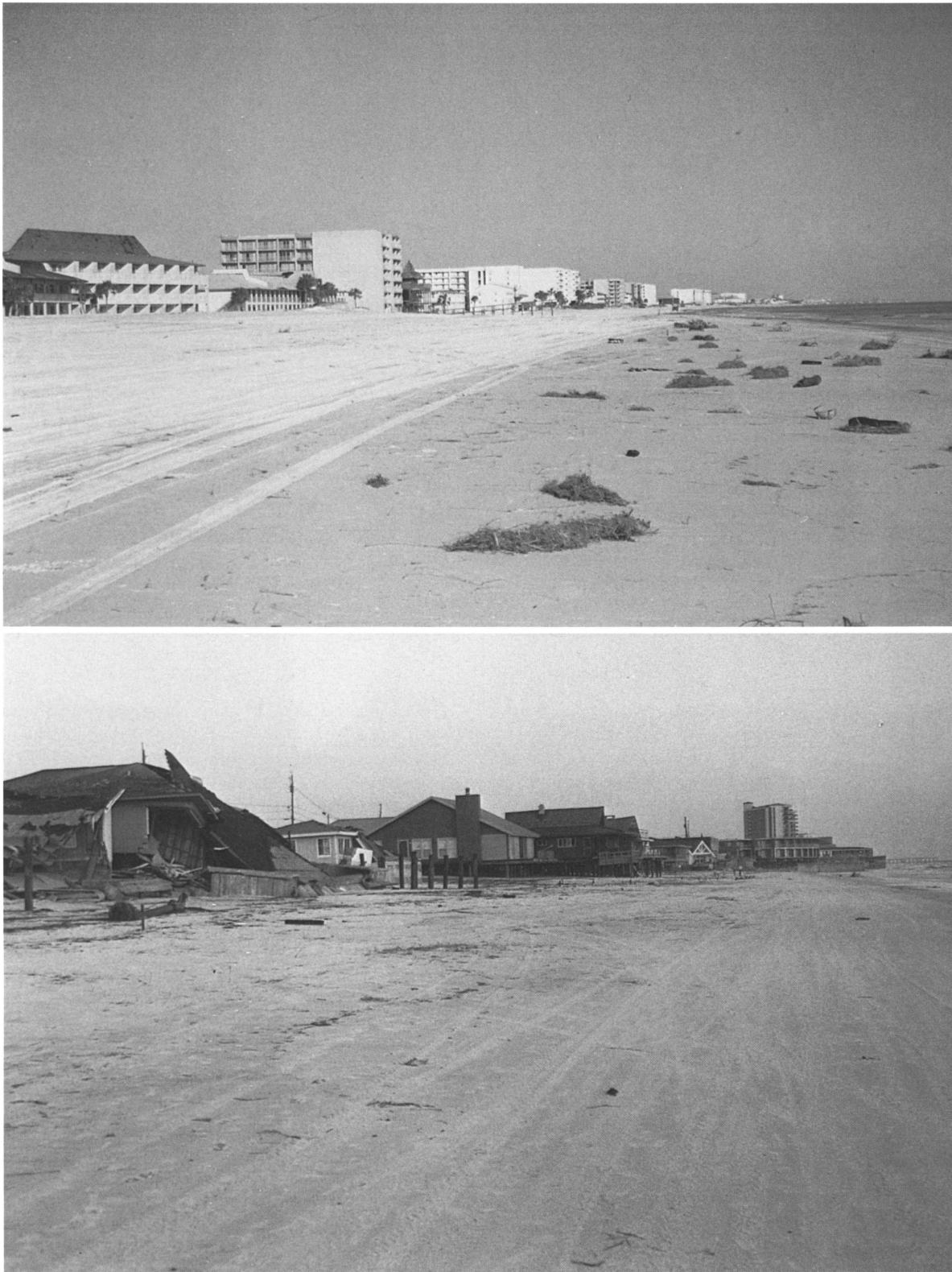
Figure 6. A. This picture from Fort Walton Beach shows the wide and flat post-storm beach. Most of the area was overwashed, leaving inland sand deposits up to 1m thick. The wide pre-storm beach and high dunes helped to reduce damage here. The large setback and immediate emplacement of overwash sand back on the beach will help mitigate against future storms. 6B. The wide, flat post-storm beach in Panama City Beach leaves all structures at a higher risk of damage by future storms. Mitigating some future damage to the single family structures in the foreground however, can be as simple as constructing an artificial dune. The seawalled structures in the background have few if any mitigation options.
