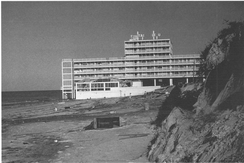
Figure 7. Erosion along Panama City Beach seriously damaged the hotel in the background. Nearly the entire structure is now seaward of the 3 m dune, with part of the building in the surf zone itself. The structure is now extremely vulnerable to even a small storm. Prevention of future damage to this structure would most likely be attempted with beach replenishment but would be only a temporary solution to the problem.
