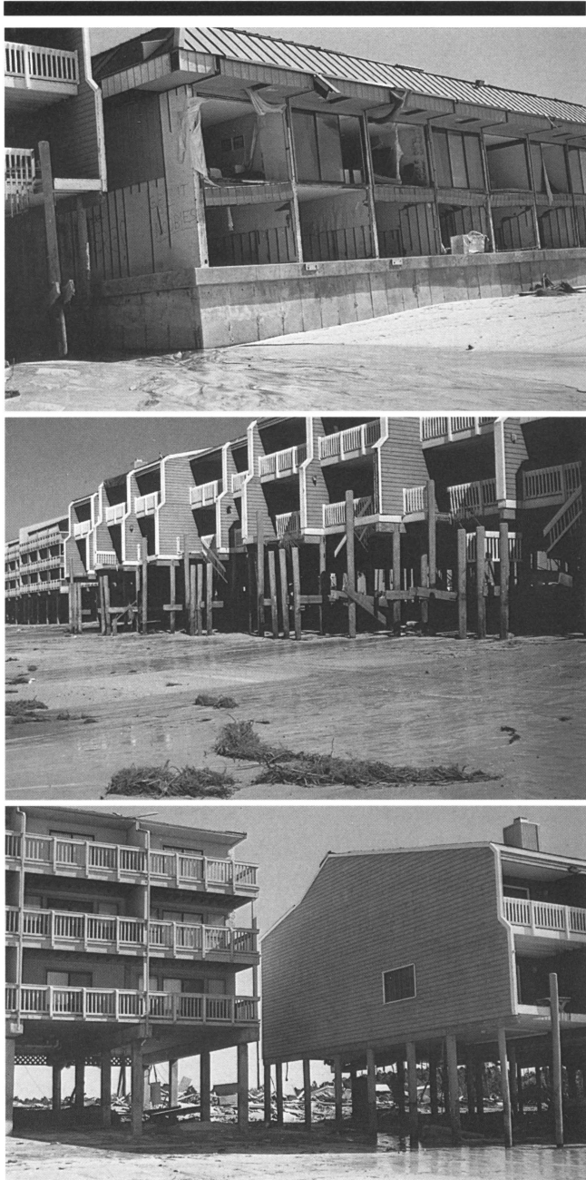
Figure 4. Three adjacent buildings in Hollywood Beach provide a basis to compare the damage mitigation capabilities of seawalls, building above grade, and building setback. Elevation and setback provided greater protection than seawalls. 4A. This building is at grade and is farthest seaward of the three. The seawall protected the structure from being undermined, but did not prevent both floors from being completely destroyed by wave action. 4B. Built approximately 3 m above pre-storm grade and set back slightly landward of the structure in Figure 4A, this building suffered minor wave damage to the first floor. The water and waves that destroyed the structure in Figure 4A passed under this building. 4C. This building (left) is set back approximately 12 m further landward and is elevated slightly higher than the structure in Figure 4B. It received no structural wave damage.
