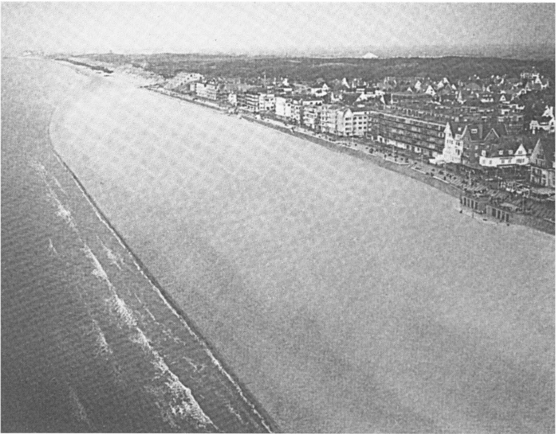
Figure 6. De Haan, Belgium, beach extension after completion of the works.
