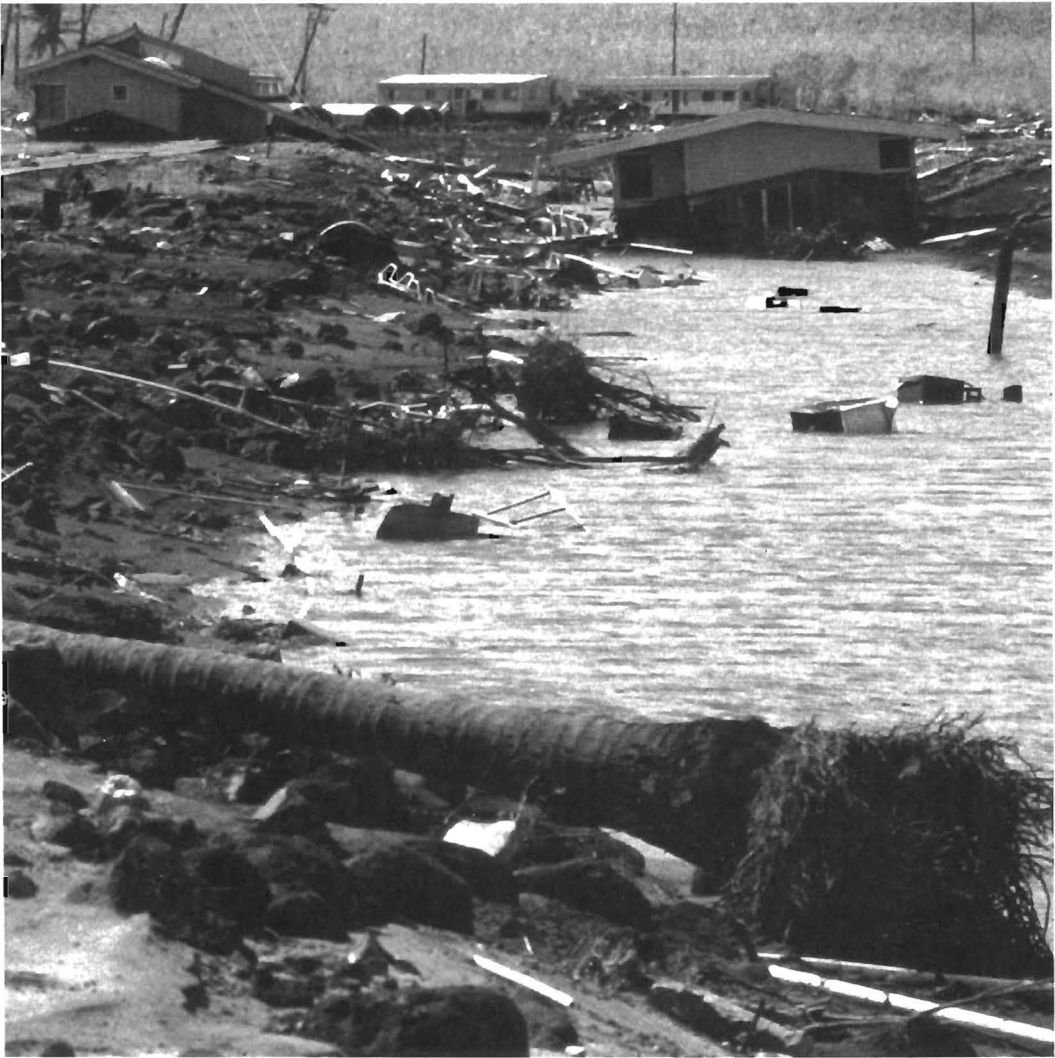
Figure 11. Overwash debris, and second and third stories of coastal dwellings located 10-50 m from their foundations. Located between Kukuilua Bay and Ka Lae Kiki Peninsula in Figure 9.
