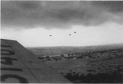
Figure 5. Nag's Head area that was flooded and overwashed.
