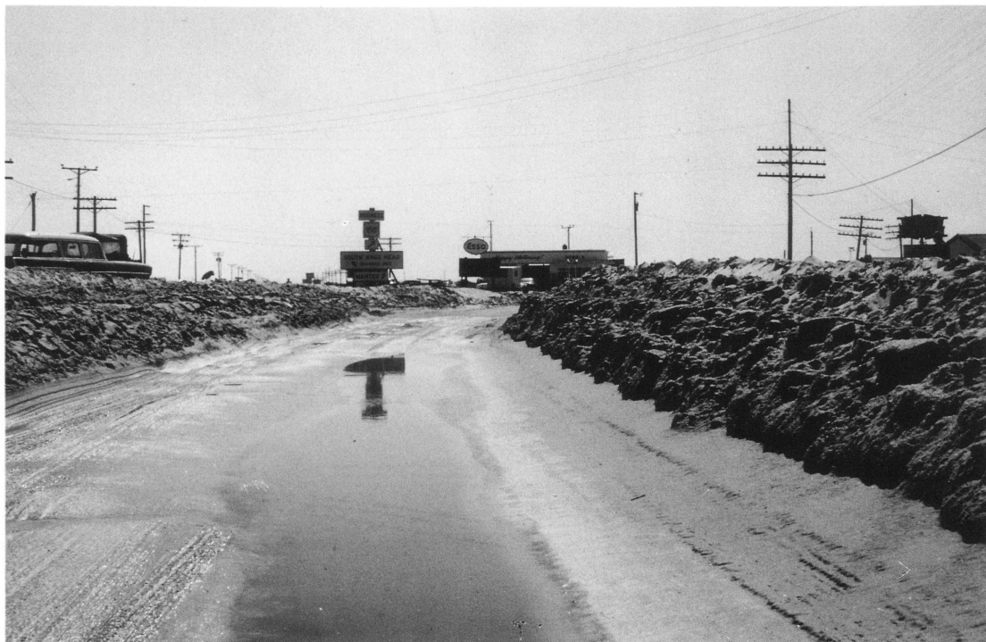
Figure 2. Overwash deposits on the road 400 feet inland from shoreline.
