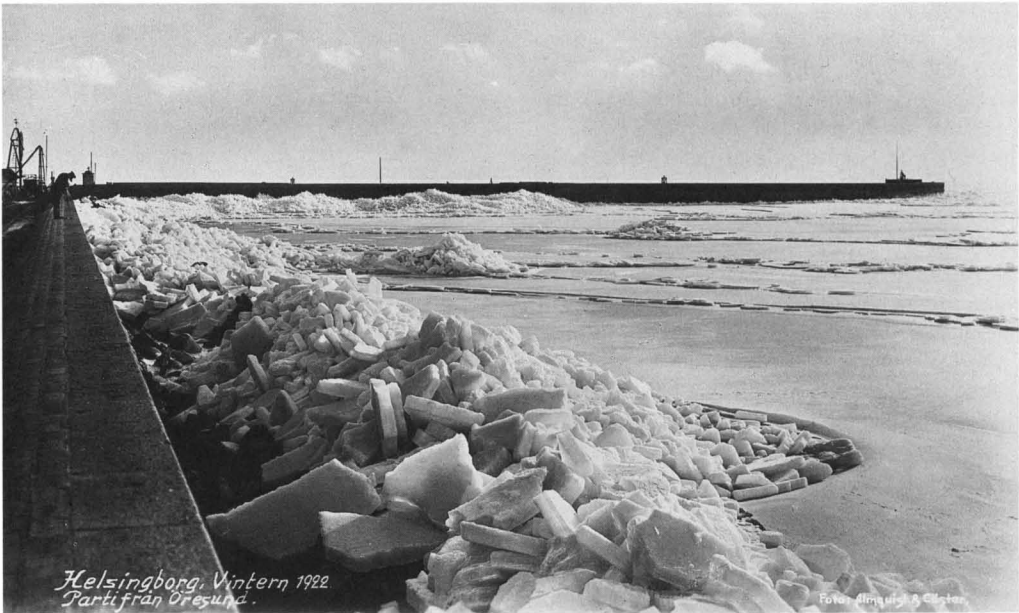
Figure 13. Minor ice pile-up at the Helsingborg, Sweden, breakwater in 1922. Photo courtesy of Swedish Meteorological and Hydrological Institute.
