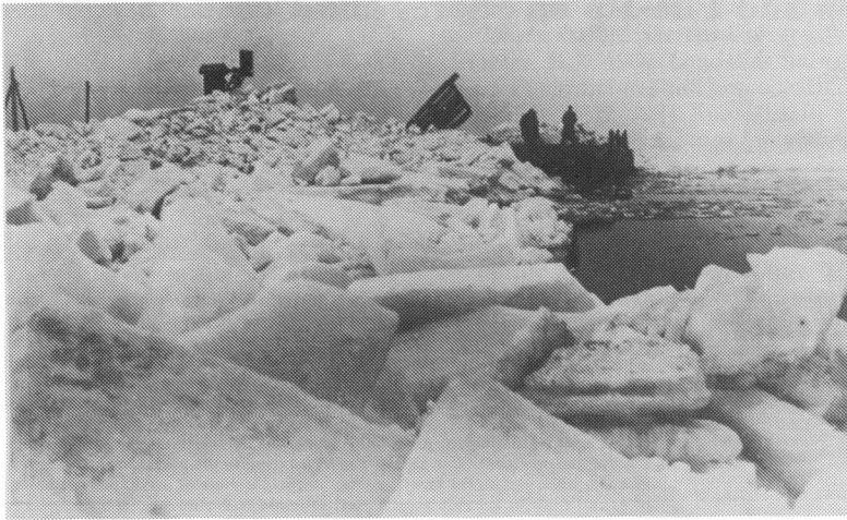
Figure 1. Ice pile-up covering the old breakwater at Knudshoved on the island of Fyn, Denmark, on 22 March 1940. This breakwater was located a few hundred meters south of the present day western landfall of the Great Belt Link. Photo courtesy of Danish Hydraulic Institute.
