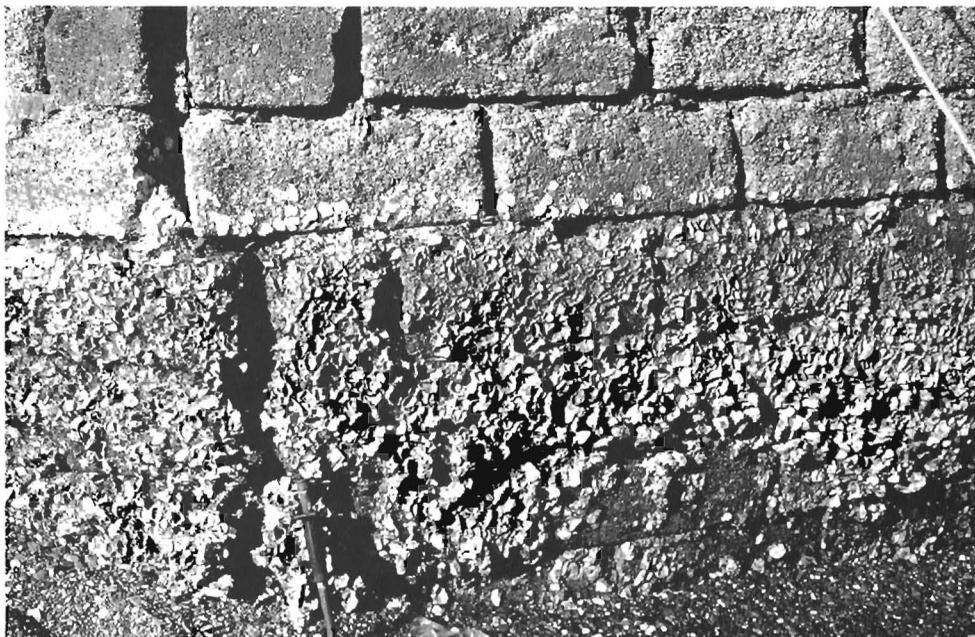
Plate 2. Example of a co-seismically elevated shoreline outside the Mediterranean region. In the Gulf of Tadjurah near Djibouti (Republic of Afars and Issas). A quay built around 1960 was uplifted about one metre in 1984 by one or several earthquakes generated by a nearby volcanic eruption. Uplifted biological sea-level is indicated by the uppermost limit of dead oysters. Level of living oysters is shown by the tool at lower left. Photograph by J. Laborel.
