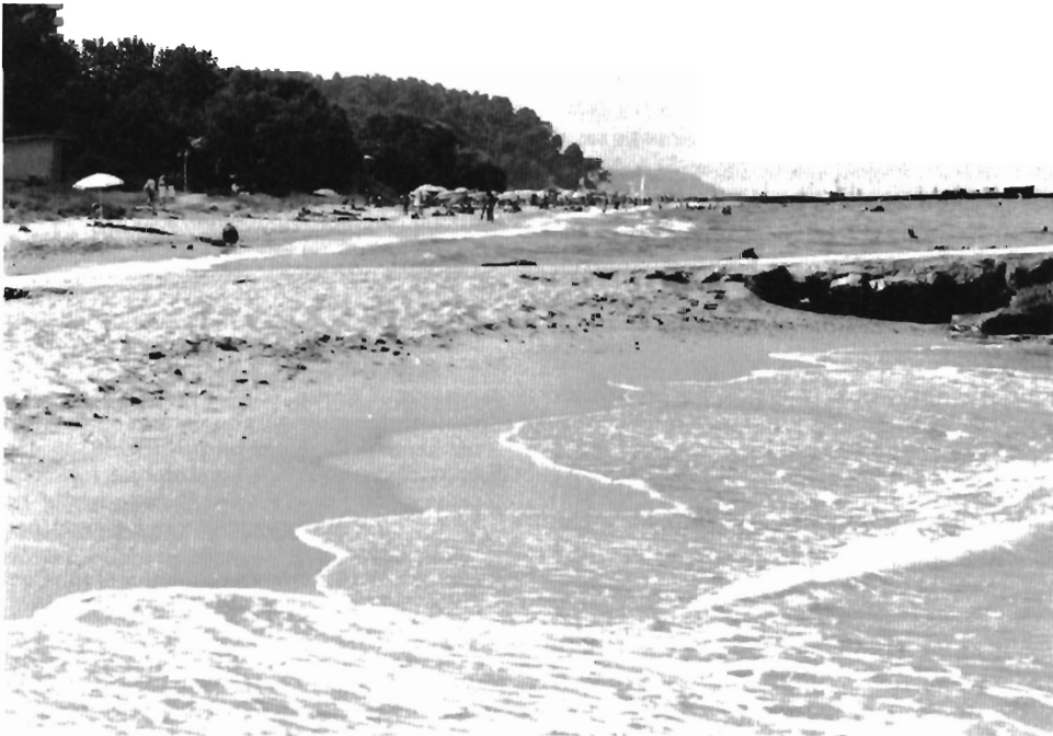
Figure 8. Kallithea Beach on the eastern coast of Kassandra Peninsula. The direction of net littoral drift (beach drift) in the swash zone towards NW is seen as an accumulation of sediment on the updrift side and erosion on the downdrift side of the jetty. Accumulation and erosion near other jetties outside the photo area are similar.
