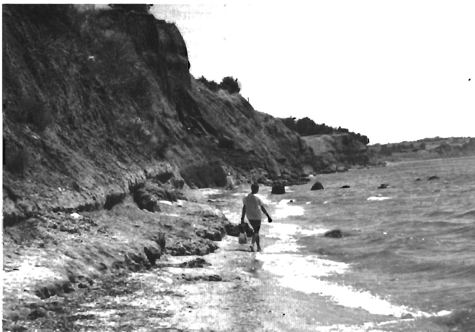
Figure 4. Coastal bluff on the southern part of Nea Potidea Beach shows evidence of strong erosion and landsliding. The bluff is of soft Mio-Pliocene deposits composed mainly of sandy red shales. The inshore slopes gently towards the sea.
