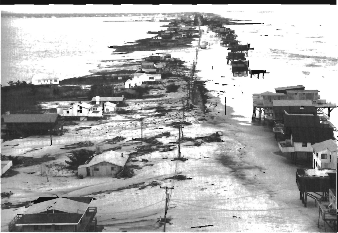
Photo 1. Dune Road in Westhampton, Long Island (New York) after the "All Hallows' Eve" northeast storm of October, 1991. Photo reprinted courtesy of Newsday /John H. Cornell Jr.
