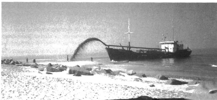
Figure 3. Nourishment by over-the-bow pumping as shown for a Danish beach, North Sea coast, 1989.
