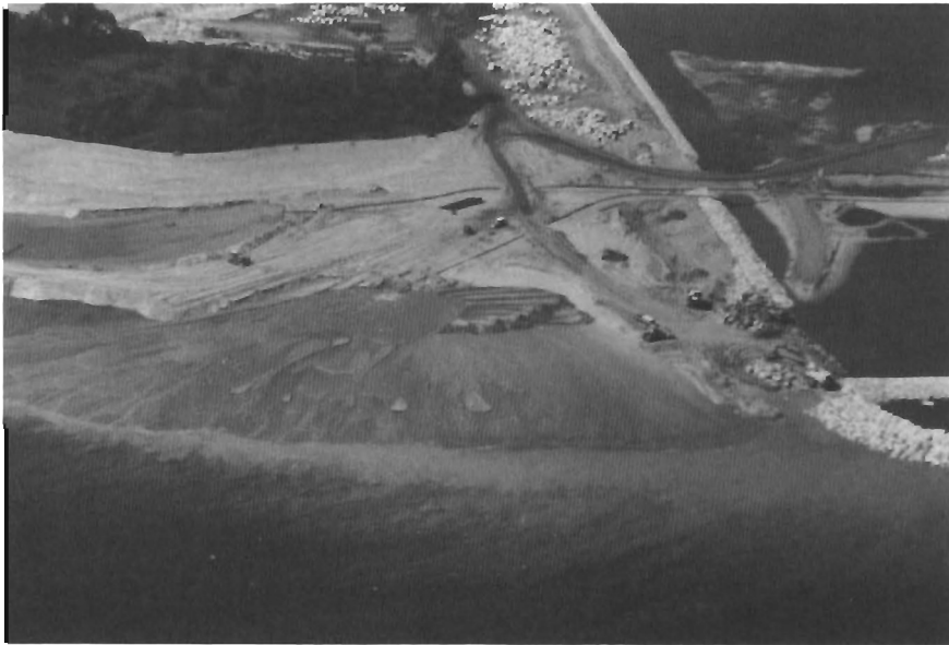
Figure 3. Aerial photograph of the fan delta taken 14 September 1988 as the fan delta was approaching maximum areal extent.
