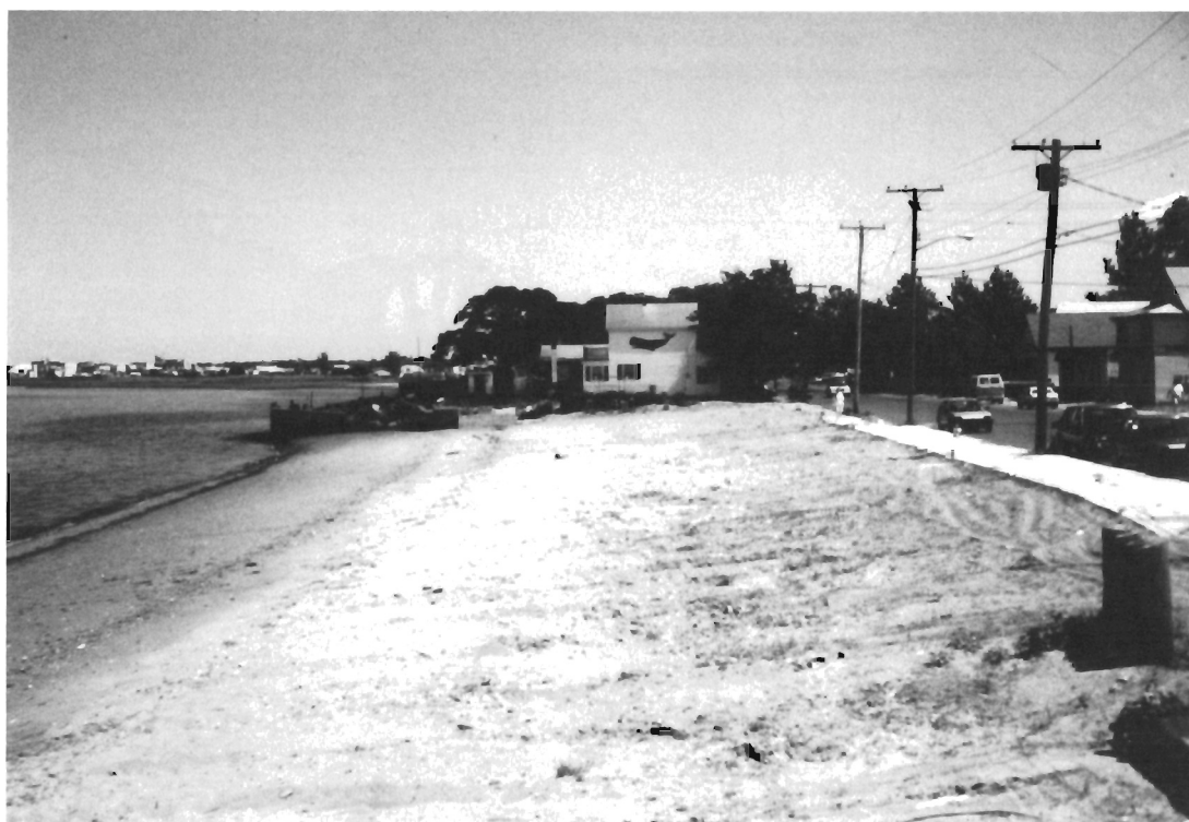
Figure 3. Union Beach, New Jersey, in Raritan Bay, facing southeast, showing the nature of bulkhead tiebacks that isolate the shoreline into compartments.
