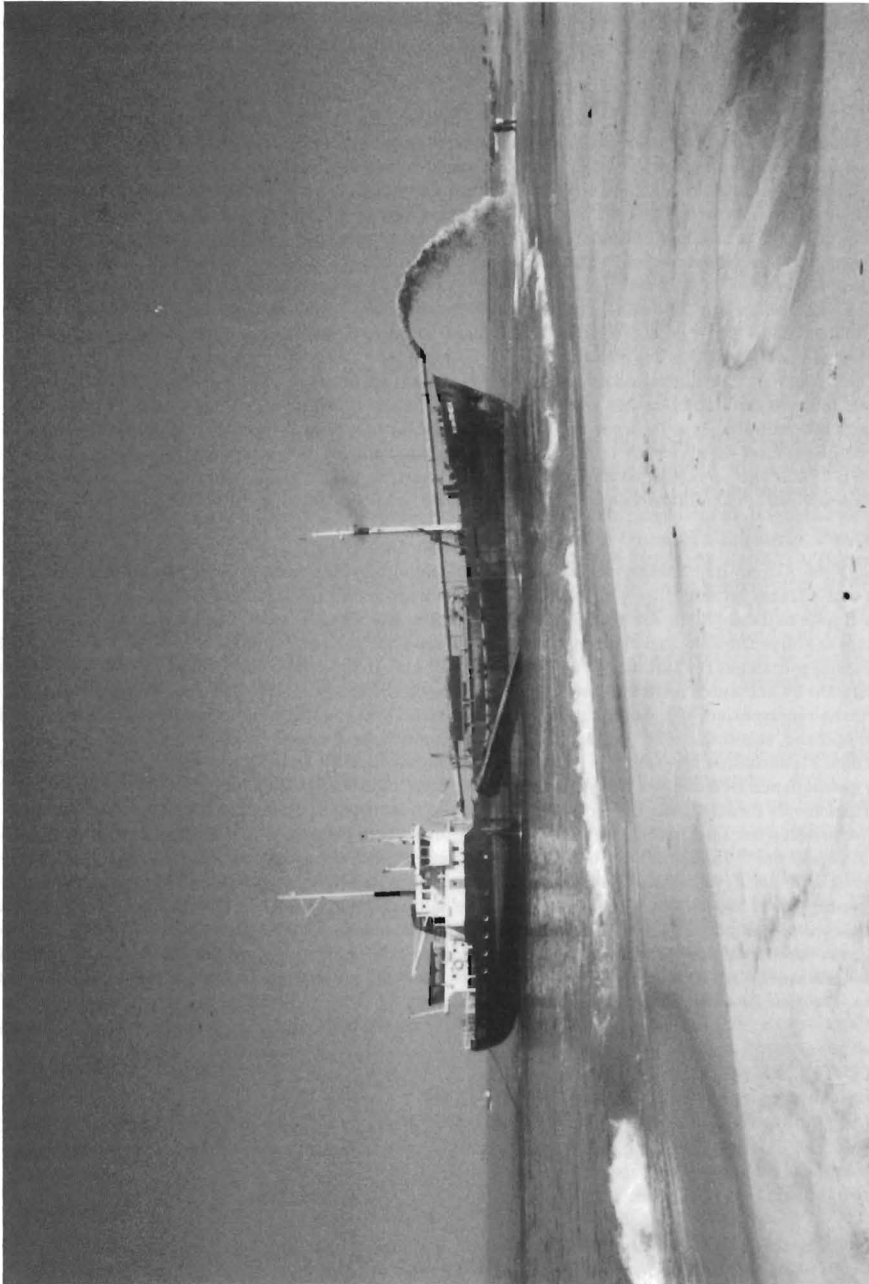
PHOTO 170. Beach spoiling on the North Sea coast. Pumping over the bow is a practical method of sand emplacement for beach renourishment projects in many parts of northern Europe. (Photo: Per Bruun, 34 Baynard Cove Road, Hilton Head, South Carolina. May 1988).
