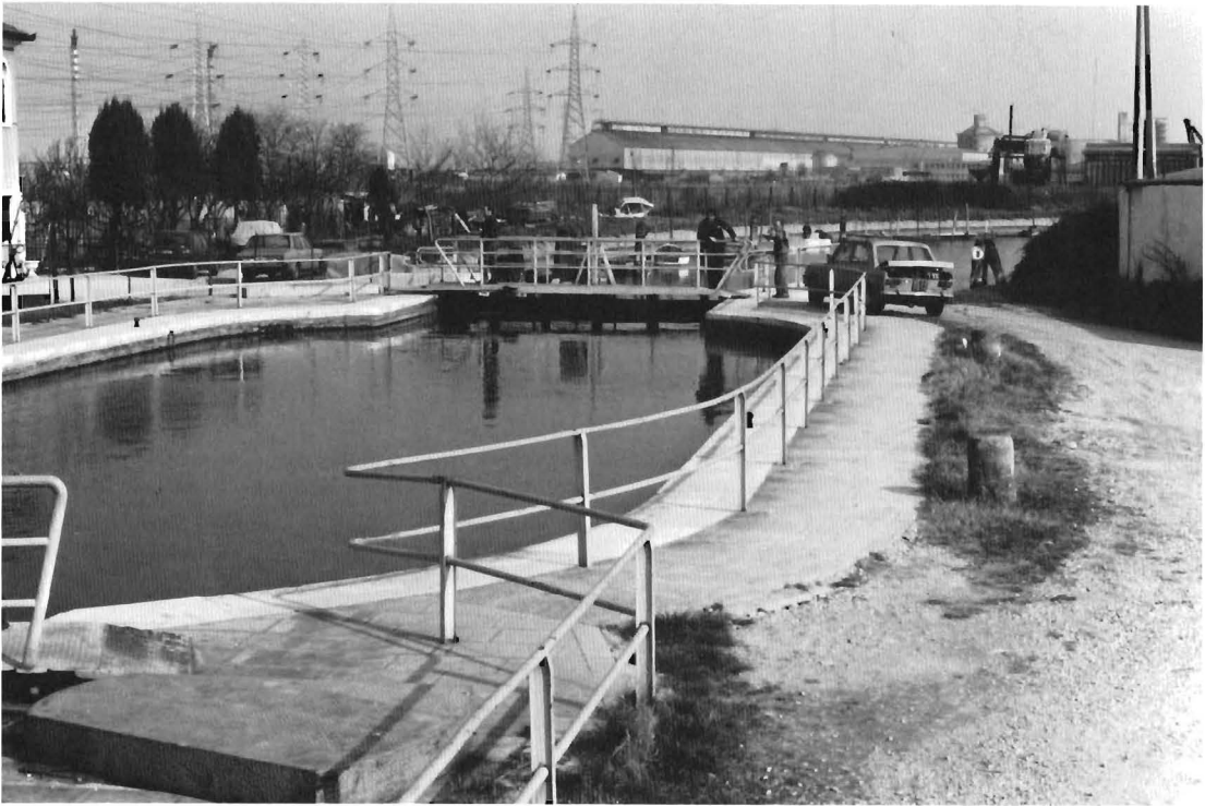
Figure 5. A small navigation lock between a freshwater course and the lagoon water (in the background) at a lower level.
