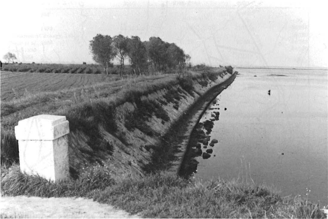
Figure 3. In A.D. 1791, six years before its fall, the Serenissima Republic delimited the landward boundaries of the lagoon by 99 cippi (boundary stones, one of which is visible in the foreground) and a continuous embankment along a perimeter of 157 km (the so-called conterminazione lagunare ).
