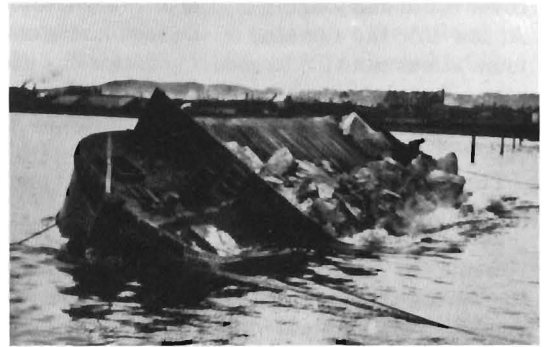
Figure 15. Construction of breakwater. Stone load being emptied.
