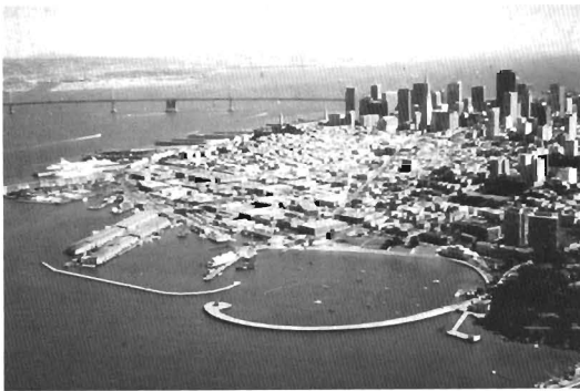
Figure 10. Aerial view of completed breakwater project at Fisherman's Wharf, San Francisco Bay, California.
