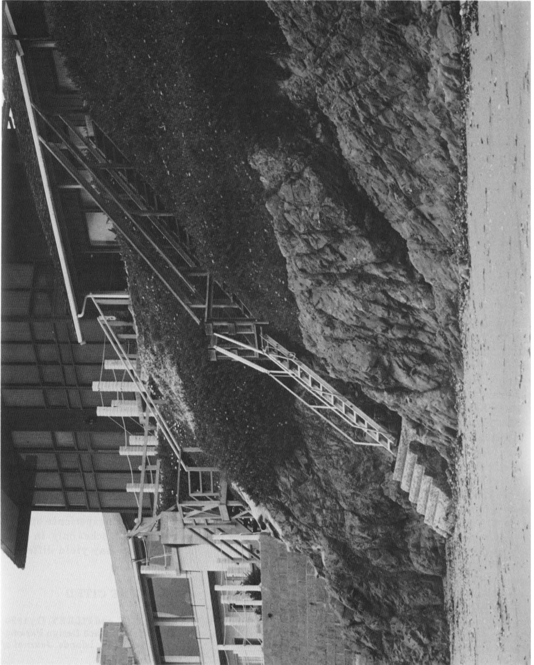
PHOTO 154. Oceanfront houses protected by seawalls and natural rocks in California. Note the variety of steps built to provide access to the beach. (Photo: H. Jesse Walker, Department of Geography and Anthropology, Louisiana State University, Baton Rouge, LA 70803).
