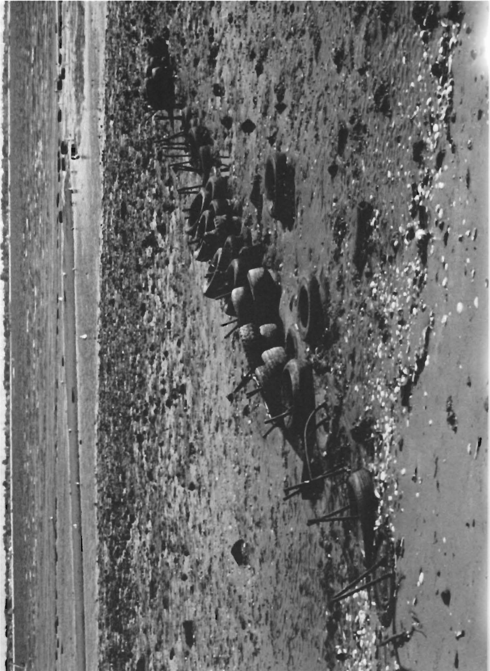
PHOTO 136. “The failed experiment.” An unsightly mess of tyre groyne on the New York shoreline. The groyne has had little or no effect on nearshore sediment distribution. Note the outer (LW) line of tyres designed to reduce wave energy at high tide. (Photo: R.W.G. Carter, Department of Environmental Studies, University of Ulster, Coleraine BT52 1SA, Northern Ireland).
