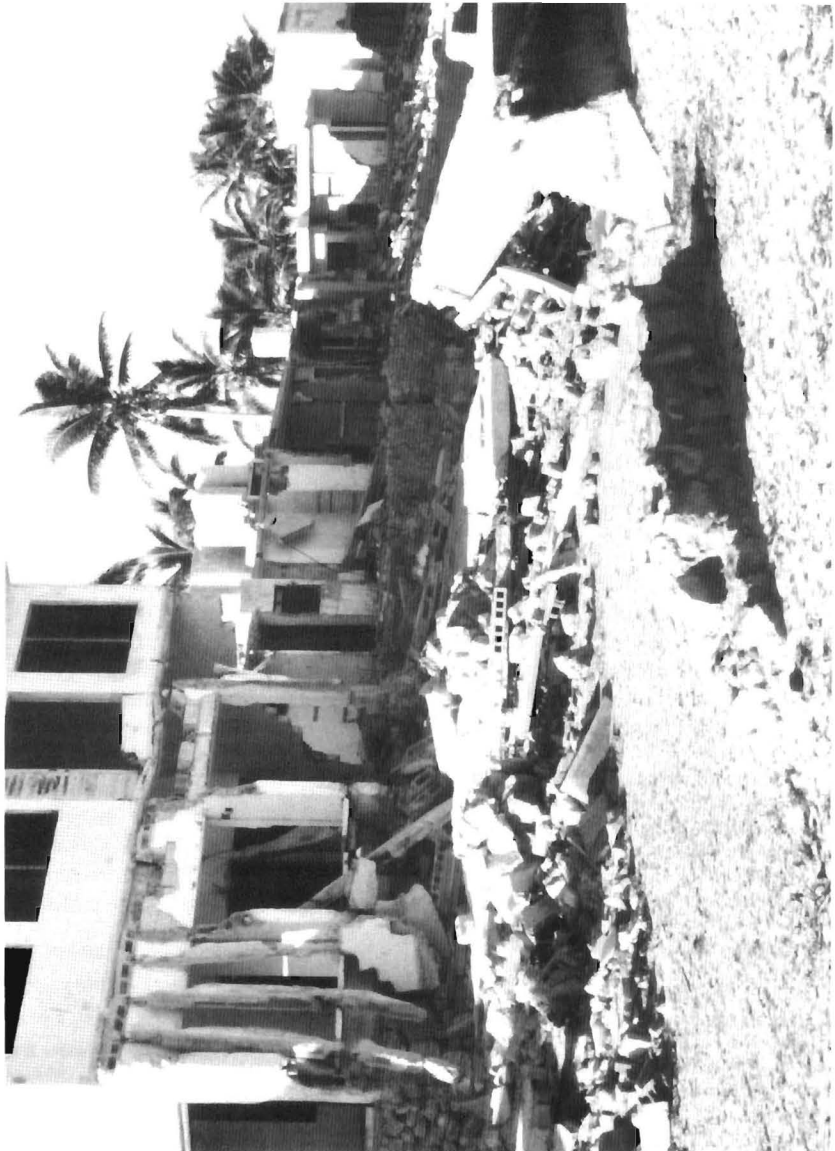
PHOTO 110. During Hurricane Gilbert in September, 1988, low seawalls at this location on the north coast of the Yucatan peninsula, Mexico were overstepped and the first row of buildings became the seawall. Seawalls can be seen in the foreground. The first row of buildings absorbed the brunt of the storm wave energy and protected the development behind them. Note that most of the debris from these concrete buildings remains in place. On U.S. barrier islands, where most small buildings are constructed of wood, flying and floating debris is a major cause of building damage. (Photo: David M. Bush, E. Robert Thieler, and Orrin H. Pilkey, Program for the Study of Developed Shorelines, Department of Geology, Duke University, Durham, NC 27708).
