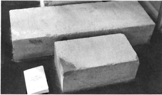
Figure 27. Concrete-weighted erosion mats form the outer periphery of the seabed-protection apron of the Eastern Scheldt barrier (illustrated in Figure 29); an 18-cm geological notebook shows scale.
