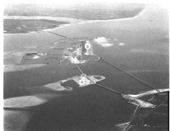
Figure 20a. The Dutch are the dredge masters of the world and frequently, as here in the Eastern Scheldt estuary, made use of artificial islands to facilitate cost-effective construction. This photograph (looking south) shows two dredged islands: (a) Roggenplaat and (b) Neeltje Jans, originally used as a construction base, and presently home of the Delta-Expo museum. See Figure 20b for further details. (Photography by Bart Hoffmeester, Aerocamera. Rijkswaterstaat Meetkundige Dienst Afdeling Reprografie).
