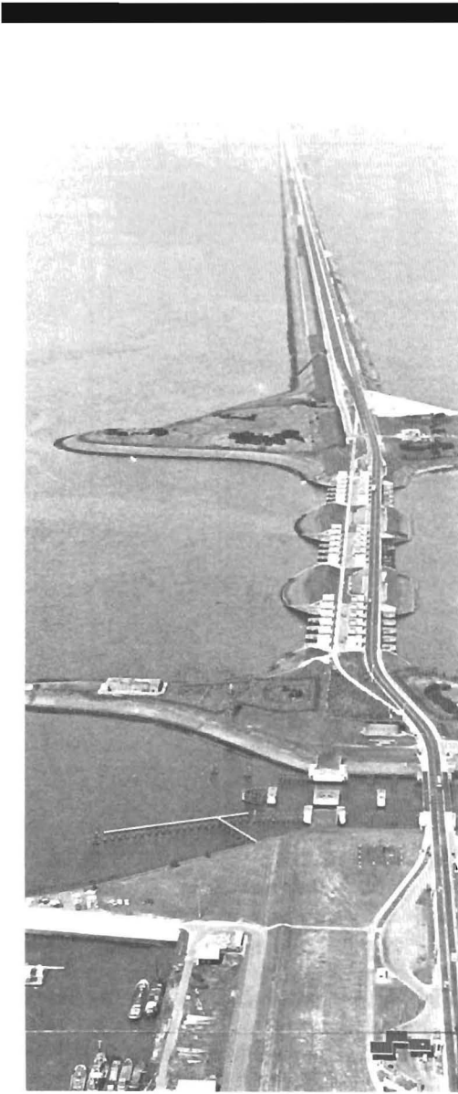
Figure 5. Air-photograph oblique of the Zuiderzee closure works. (Photograph courtesy of Bart Hofmeester, Aerocamera. Rijkswaterstaat, Meetkundige Dienst Afdeling Reprografie).
