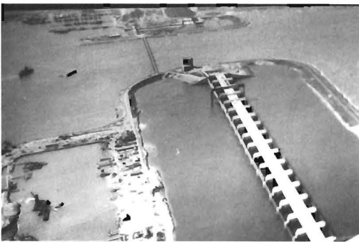
Figure 21b. Following completion of the Haringvliet sluice-gate barrier, the cofferdam was flooded and subsequently dismantled. (Rijkswaterstaat Meetkundige Dienst Afdeling Reprografie).
