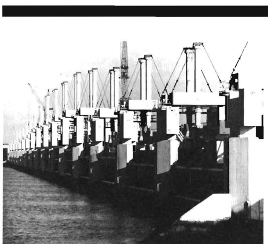
Figure 33 cont. (c) A close-up of the pier-supported, lift-gate sections of the barrier.
