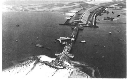
Figure 17. Veerse primary-embankment barrier showing: (a) tugs positioning the last caisson for the "sudden closure" core of the dam. (b) The approach embankment with a crest road; this will eventually extend over the caisson core. (Photography by Bart Hofmeester, Aerocamera. Rijkswaterstaat, Meetkundige Dienst Afdeling Reprografie).
