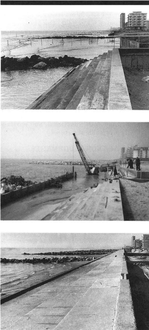
Figure 8. Chaotic situation along western stretch of Lido di Jesolo in December 1966 (above), during construction of defences (centre), and when nearly completed in 1970 (below).
