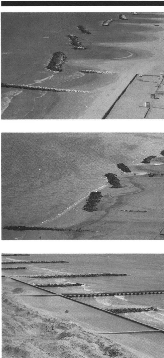
Figure 10. Effects of breakwater reefs: beach in 1977 (top) and 1987 (centre). Defences perpendicular to shoreline (bottom) are ineffectual and frequent artificial renourishment is necessary.
