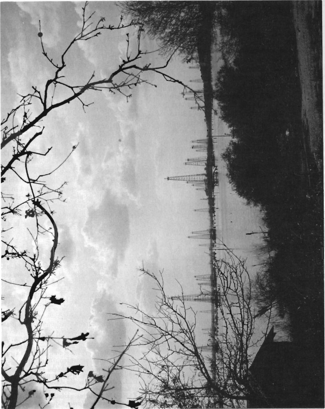
PHOTO 134. Evidence of subsidence in the oil field at Baytown, Texas. The small islands between the derricks are shell middens. (Photo: H. Jesse Walker, Department of Geography & Anthropology, Louisiana State University, Baton Rouge, LA 70803).
