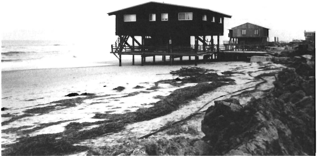
Figure 1. Beach home at Sandbridge Beach, Virginia, in "imminent danger of collapse." This photo was taken soon after the storm of March 7-11, 1989.
