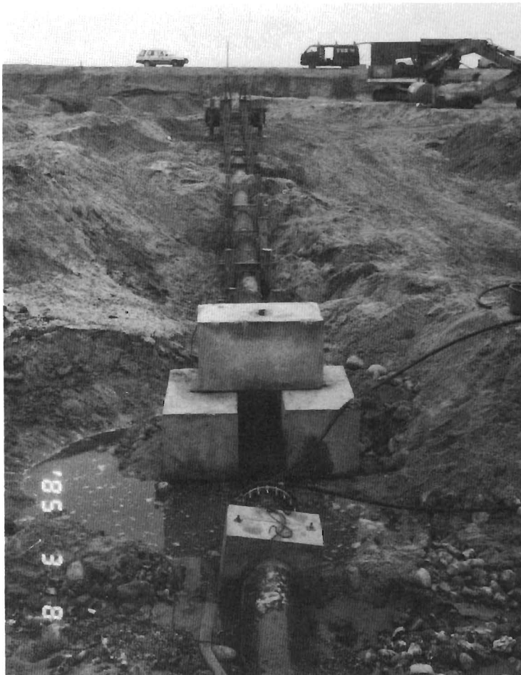
Figure 2(b). The land-end of the shore-pipe under construction (1985). (Danish Coastal Directorate).
