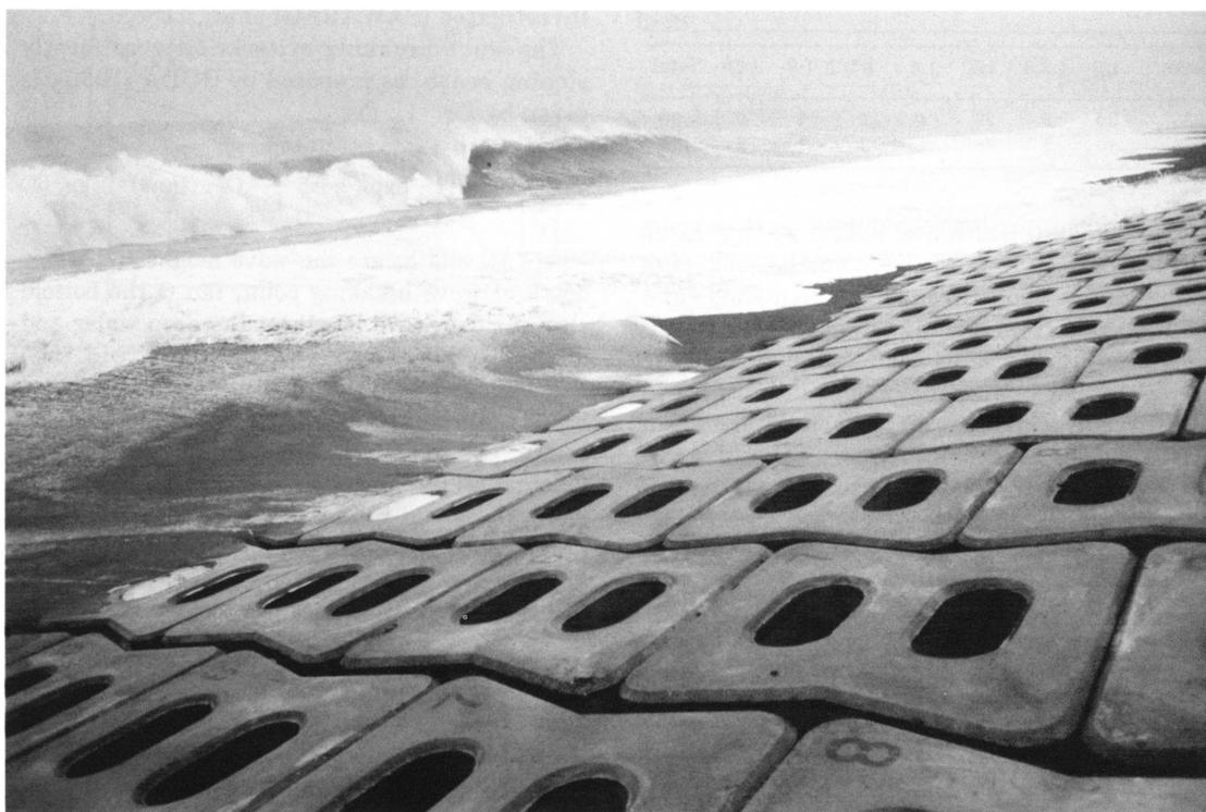
Photo 1. An example of a sea dike of gentle slope constructed in Japan.
