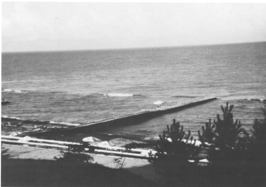
Figure 3. Coastal protection structures at Sochi (Photo: M.L. Schwartz).
