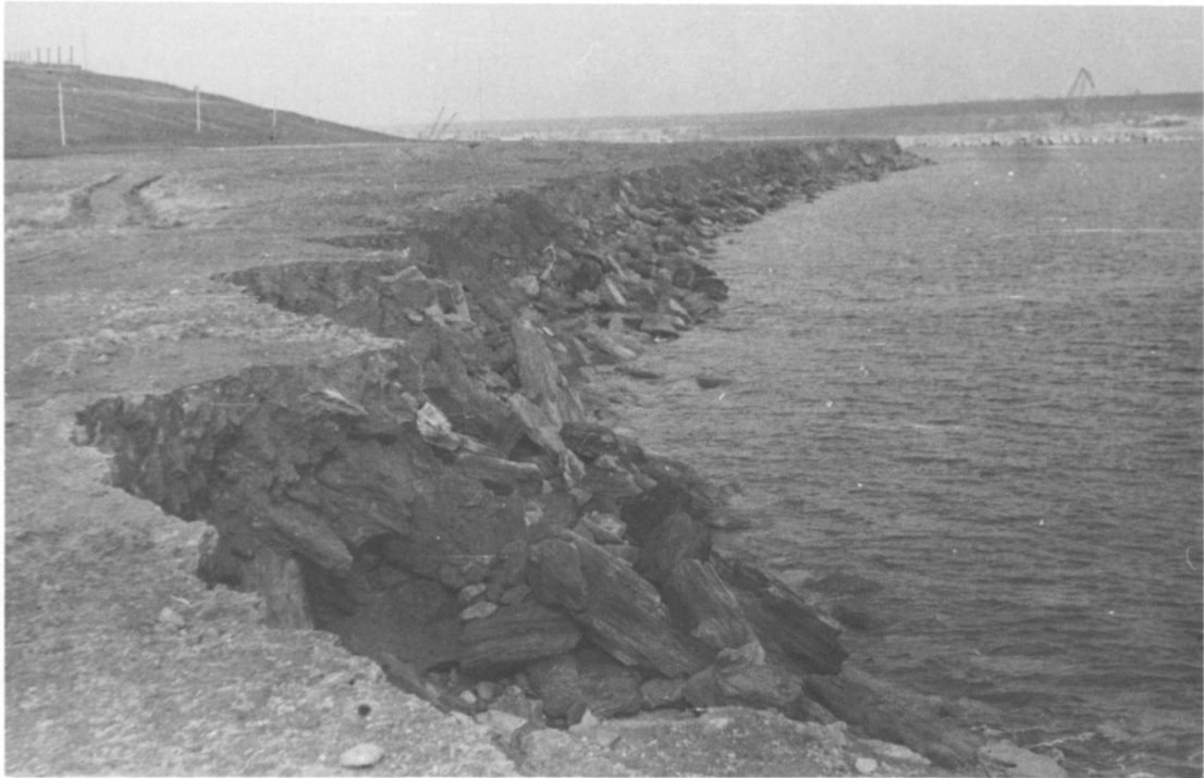
Figure 5. Embankment built in front of cliff site shown in Figure 4 (Photo: Y.D. Shuisky).
